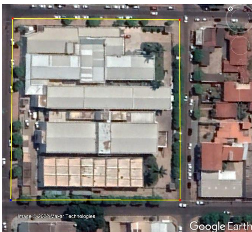
Figura 8 - Hospital Regional de Rondonópolis (HRR)
